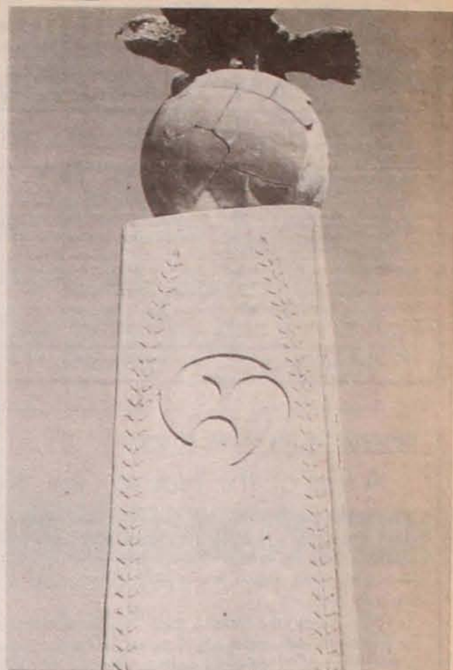
TOP DETAIL to MONUMENT 'A' Ornament at top of monument dedicated in 1944. Beak and face of eagle are damaged, sections of the globe have cracked off.
