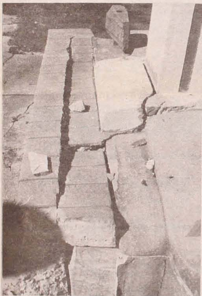
DAMAGE TO MONUMENT 'B' Tread on south side of tank is badly cracked.
