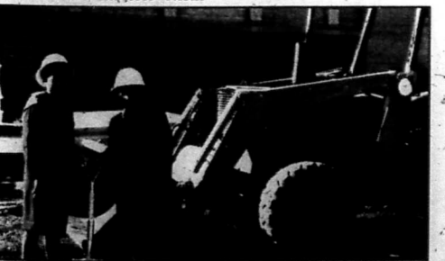
LITTLE TOKYO'S NEW DIGGINGS—City Councilwoman Rita Walter (right) and JANM executive director Irene Hirano stand over the spot where ground was broken for an 85,000 square-foot "Phase 2 Pavilion."
