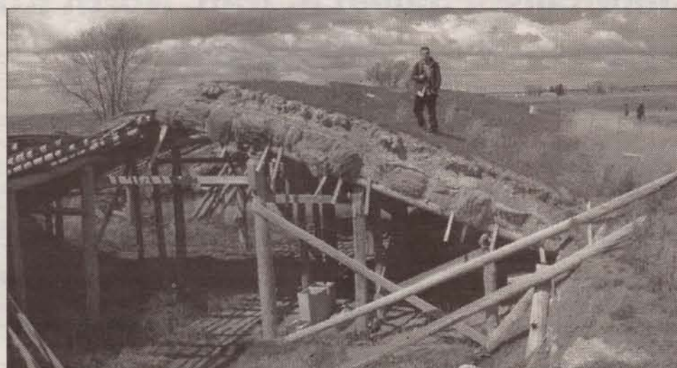
University of Oregon Architecture Student Edwin Stanculescu on the roof of the root cellar at Minidoka. This semi-underground structure, built by internees along local lines, was used to preserve vegetables they cultivated themselves in the surrounding fields to feed the more than 10,000 Japanese Americans incarcerated at the camp between 1942 and 1945.
