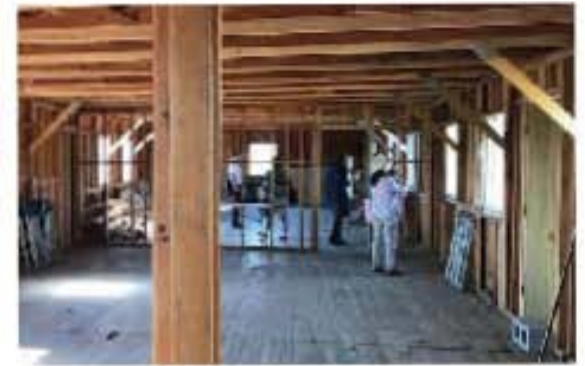
A barrack interior with a dividing wall
